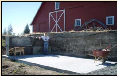
Manure Storage Structures
